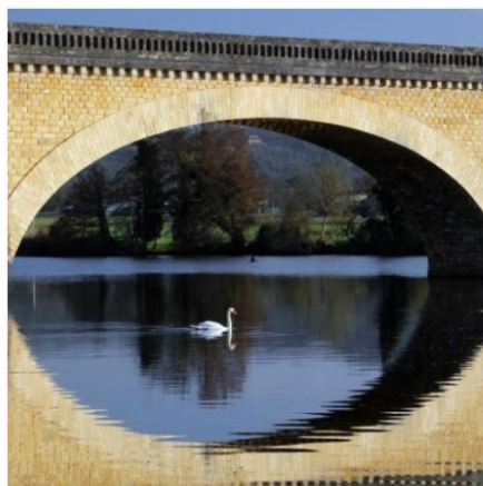
Mauzac railway bridge (DL)
